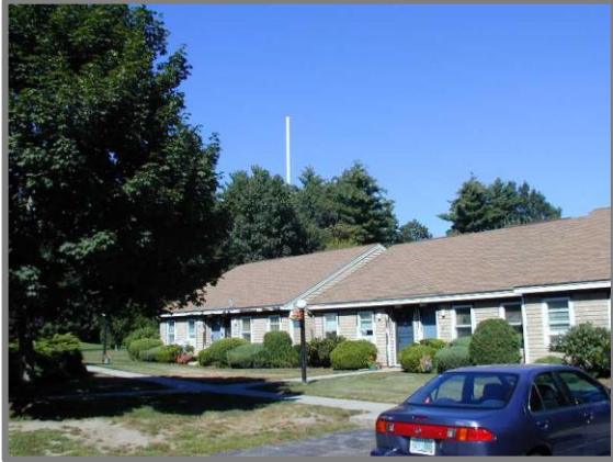
Figure 6: Flush-Mounted Monopole in Bedford, NH
