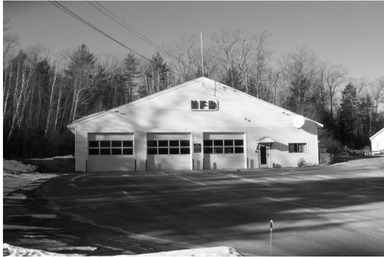
Figure 1 - Town Fire Station
