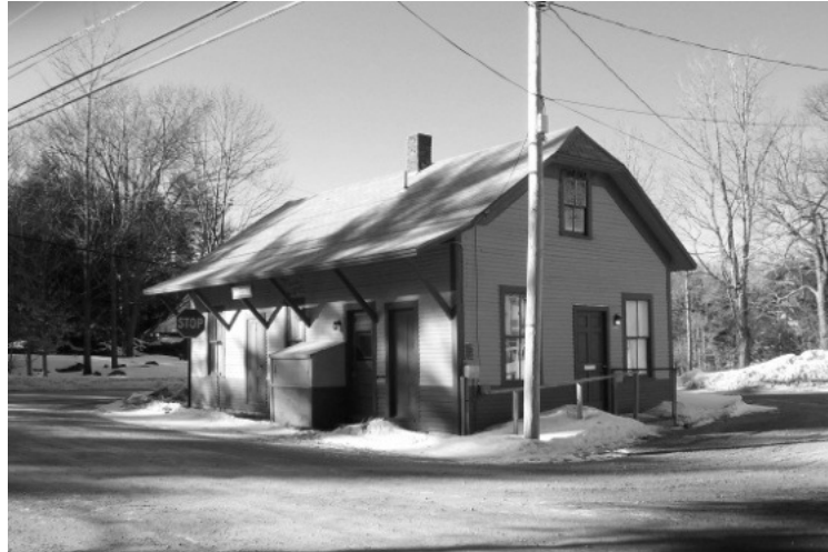
Figure 3 - Town Police Station
