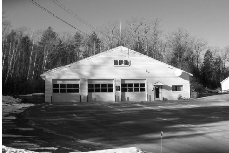
Figure 1 - Town Fire Station
